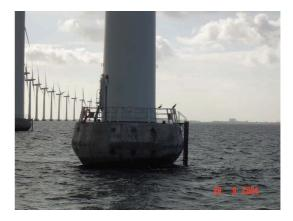
*Figure 9:* The access ladders for smaller boats are damaged after winters with ice. A special weak link is build into the ladder in order to limit the damage.
