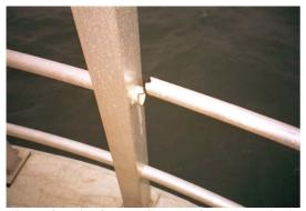
*Figure 8:* The distance between the posts in the fence has been too large creating vibrations caused by the wind. The repair is simple.
